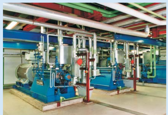
MC 80-260, 13 stages, Head 1360 m, Capacity 100 m 3 /h, 517 kW
