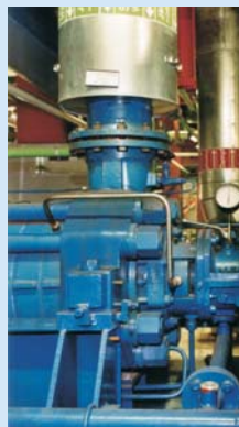
MC 80-260, 13 stages, Head 1360 m, Capacity 100 m 3 /h, 517 kW
